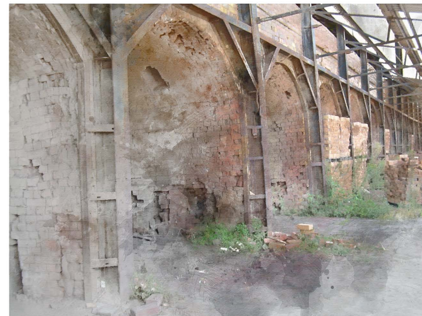
DECOMMISSIONED BRICK OVEN
