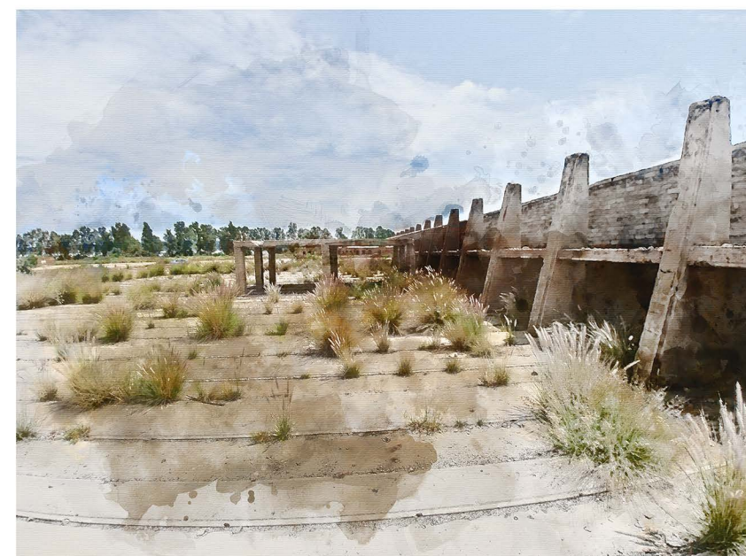
LEFTOVER BRICK DRYING TRACKS
