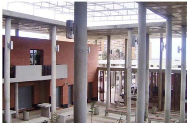
Fig. 5-102. Baragwanath Transport Interchange atrium (Adopted by Author 2018)
