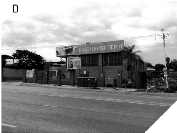
light industrial along Vom Hagen st: by author 2018
