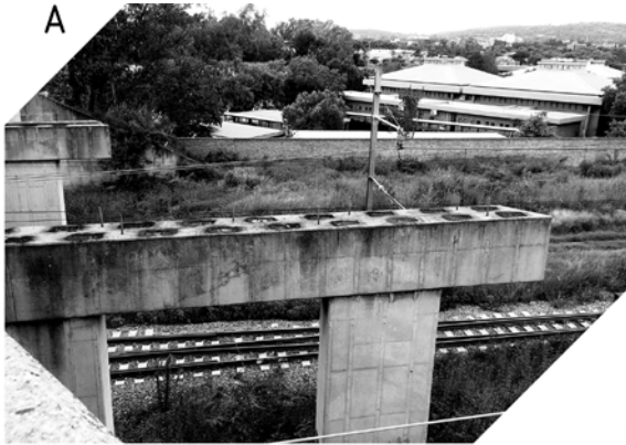
Rail Bridge structure: by author 2018
