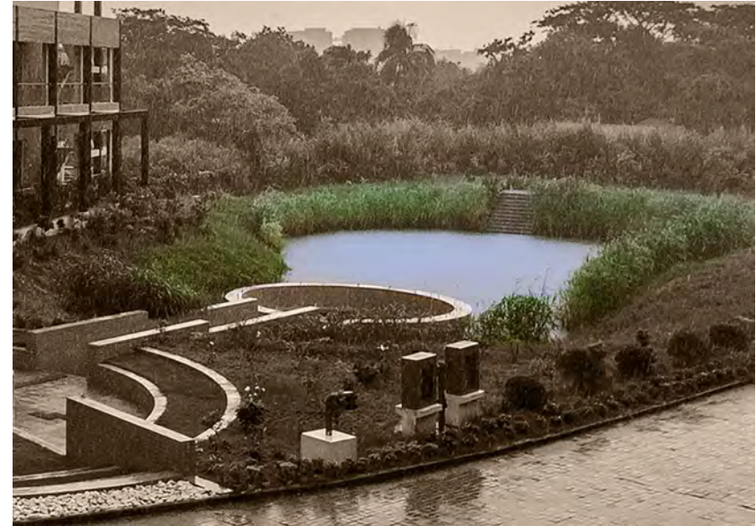
Figure 4.11 - Image showing a retention pond that is used to store rainwater to be used as greywater in the adjacent building and irrigation water for the surrounding landscape (Plummy-fashions.com, 2018).
