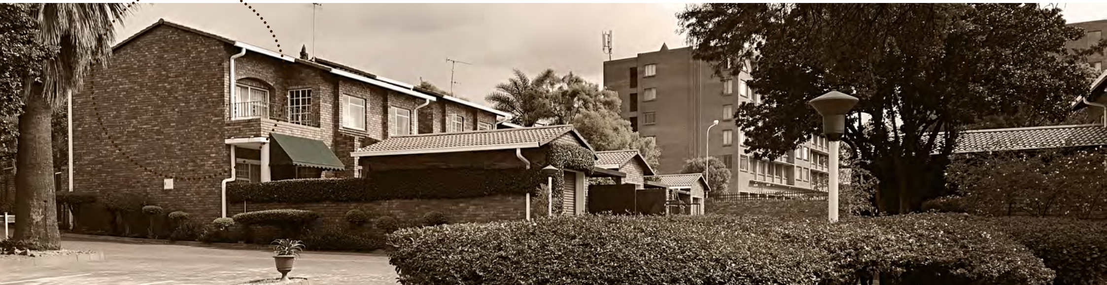
Figure 3.13 - Photograph indicating the excessive use of face brick in Centurion (Photograph taken and edited by author, 2018)
