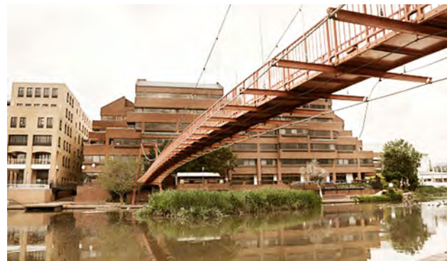
Figure 3.52 - Pedestrian suspension bridge connecting the businesses with the public park (Author, 2018).
