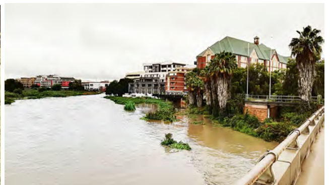
Figure 3.62 - Centurion Lake (photograph taken from Hendrik Verwoerd Drive) during a flooding event (Author, 2018).
