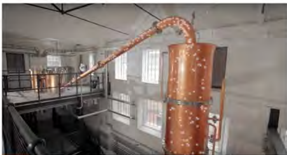
3 Rectifying Column: Distilling process
