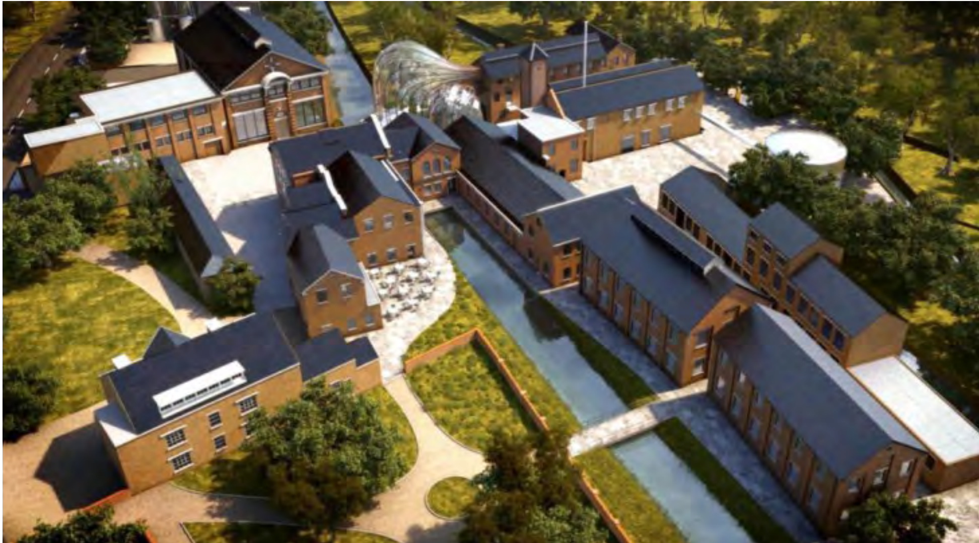
Figure 5.21 - Laverstoke Mill after the completion of the restoration project to convert the mill into a gin distillery for Bombay Sapphire Gin (Bombay, 2014). © University of Pretoria
