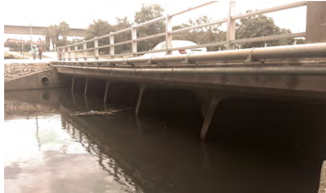
Figure 3.58 - Vehicular bridge with Lenchen Road running over the river. The bridge's structure creates the entrance channels for incoming water to the lake (Author, 2018).
