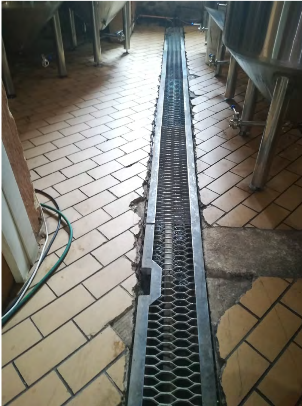
Figure 5.38 - Photograph of the recessed gutter, located within the distillery to ensure that any leakages are removed from the space (Author, 2018).
