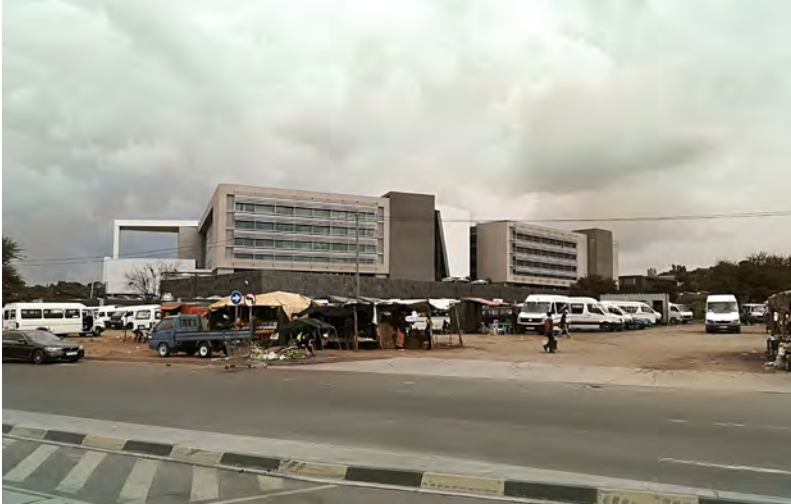
Figure 3.27 - The new (2017) BCX building surrounded by informal markets and taxi ranks (Photograph taken and edited by author, 2018).
