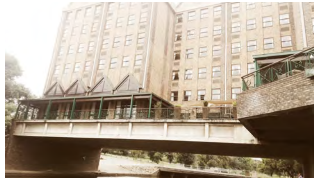
Figure 3.55 - Centurion Lake Hotel; suspended over the Hennops river by using large concrete beams (Author, 2018).
