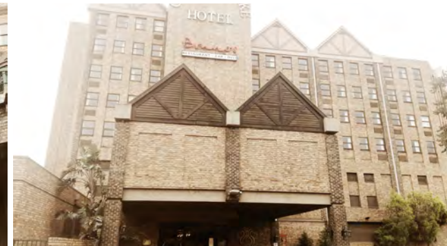
Figure 3.56 - Centurion Lake Hotel's entrance facing south, away from the Centurion Lake to the north (Author, 2018).
