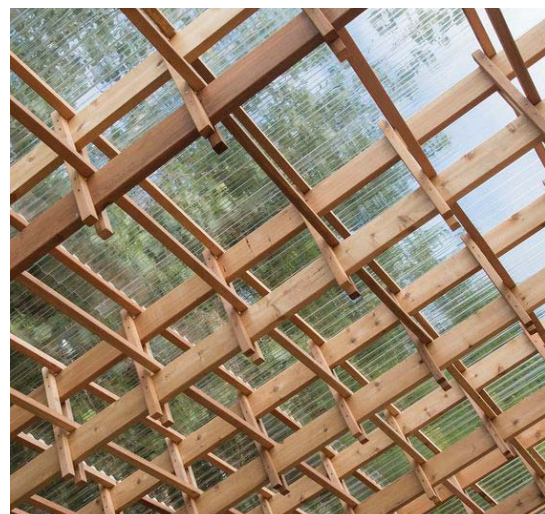
Figure 8.8. Sticks Roof Structure (Architizer, 2016)
