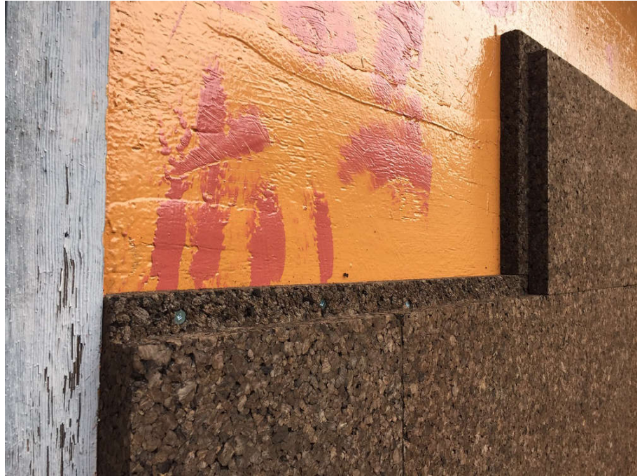
FIG. 129 ;THERMACORK FACADE (THERMACORK, 2018)
