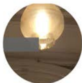
Interior Ceiling Fixture: Original suspended light fixture in the main entrance.
