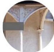
Pillars: The turned timber pillars are from apart of the original structure.
