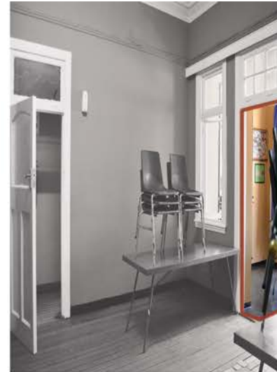
Room 1: The double doors through the house have been removed. The door frames and decorative trims remain.
