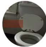
WC: The water closets have been replaced throughout the house.
