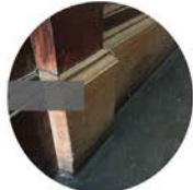
Skirting: The skirting is the original solid meranti .
