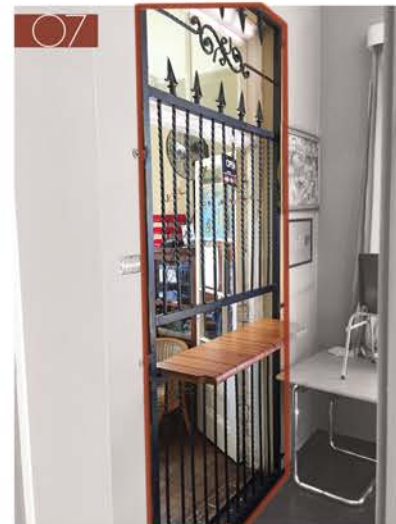
Room 2: The door from room 2 to 3 was replaced with a security gate in order to isolate the office.
