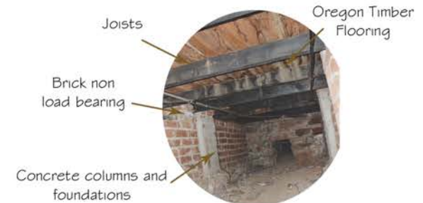
Suspended timber floor
