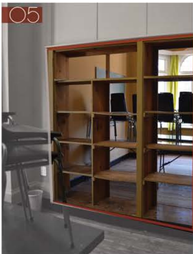
Room 5: The BIC that separates the two rooms is the original. The doors were stolen. Figure 31: Interior Analysis (Author 2018)
