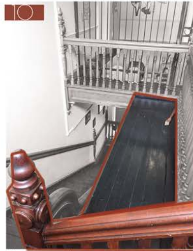
Staircase: The staircase is a combination of the original balustrades with alterations to the missing connections. The tread, rise and landings have been painted.
