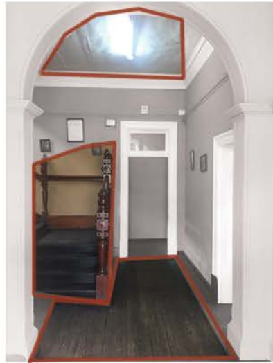
Foyer: The floor and staircase have been altered. Parts of the kiaat staircase are original as well as parts of the Oregon pine floor are originals. The decorative ceiling
