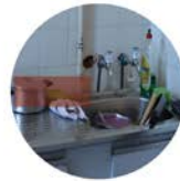
Sink: All kitchen sinks have been replaced with intergated kitchen sink tops.
