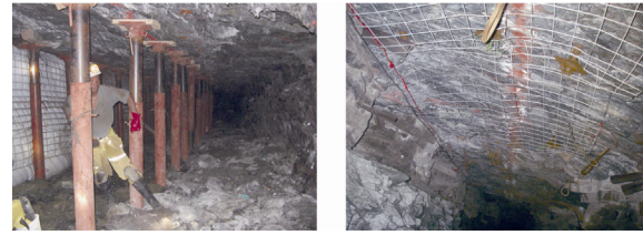
Fig. 8. Examples of support in deep gold mines prone to seismicity.
