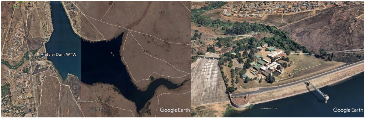
Figure 6-5: Location and aerial view of the Rietvlei WTW.
