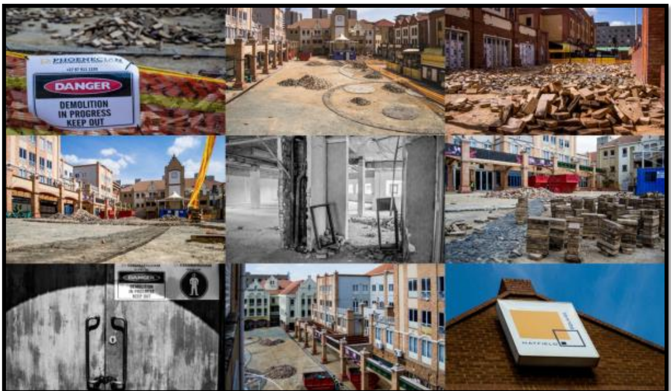
Figure 4: The demolition of Hatfield Square
