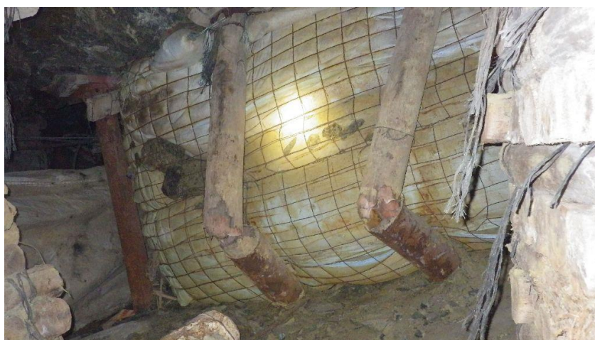
Fig. 10. a) A barricade of a sandfilling paddock as described in 1946 (after Jeppe 16 ) and b) a modern filled backfill paddock. Note how the elongates buckled owing to the large amount of convergence in the back area and the bulging of the backfill bag (photograph D.F. Malan).
