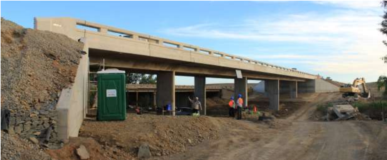
Fig. 2. Van Zylspruit integral bridge towards end of construction
