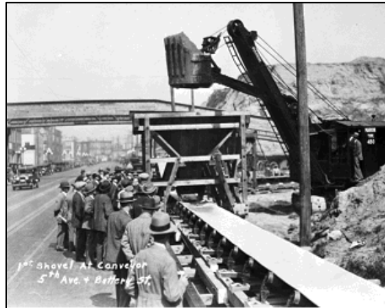
Figure 1.1: One of the first conveyor belts used in the mining industry (Habasit, 2011)
