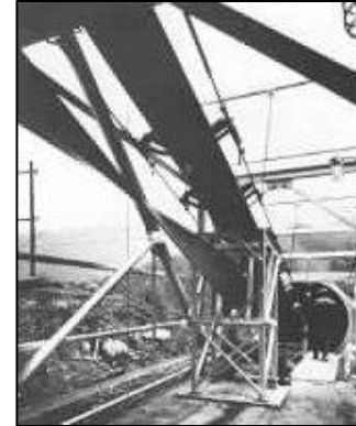
Figure 1.3: Implemented Turnover Conveyor Belt (Darling, n.d.)
