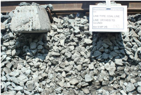
Recycled Ballast Sample "A" at Km 9
