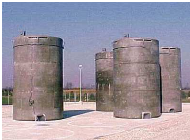
Figure 1.2: An image showing dry casks placed on concrete pads. Taken from reference [3].
