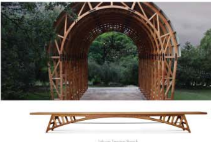
The trusses of the Chapel and joint details by Dawid Krynauw are crafted so that structural elements can become an exposed feature (images from www.davidkrynauw.com ).
