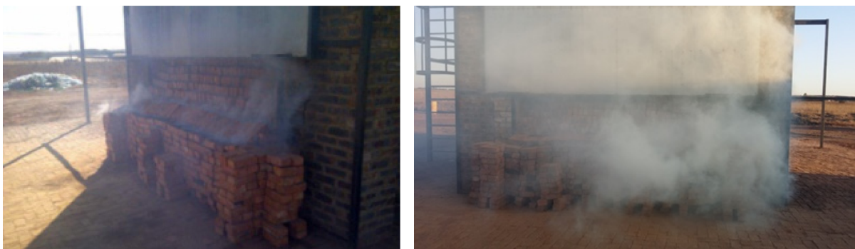
Figure 42: Visible smoke exiting the semi-enclosed sideboards during kiln start-up
