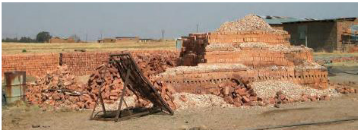
Figure 18: Typical informal clamp kiln (Cermalab, 2014)
