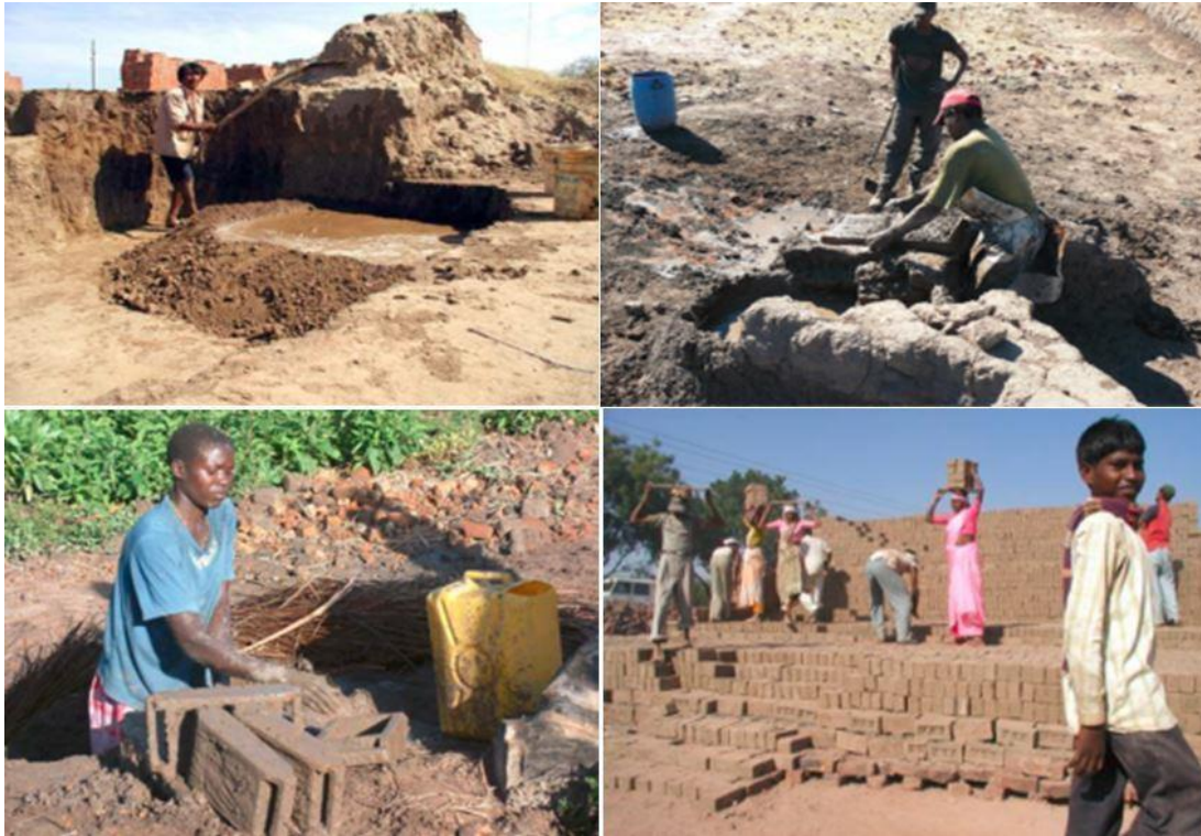
Figure 20: Typical brick making activities in informal sectors in Asia and Central America (Cermalab, 2014; Goyer, 2006)
