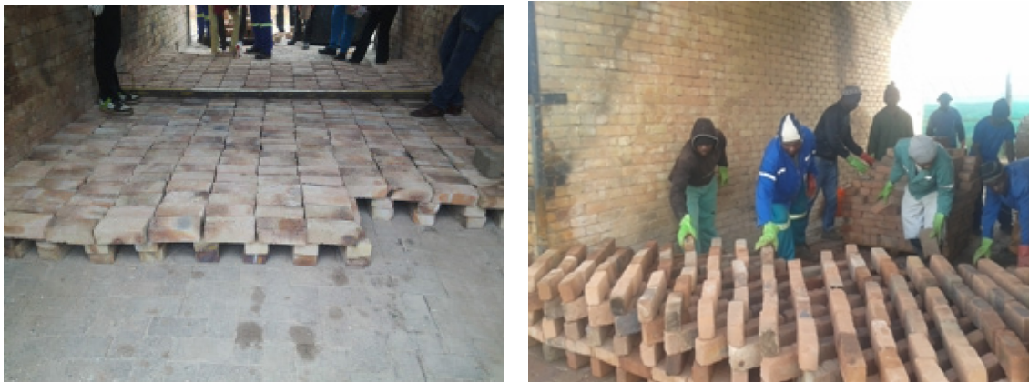
Figure 38: Construction of 'table' (left) and 'scintle' (right) inside the model kiln
