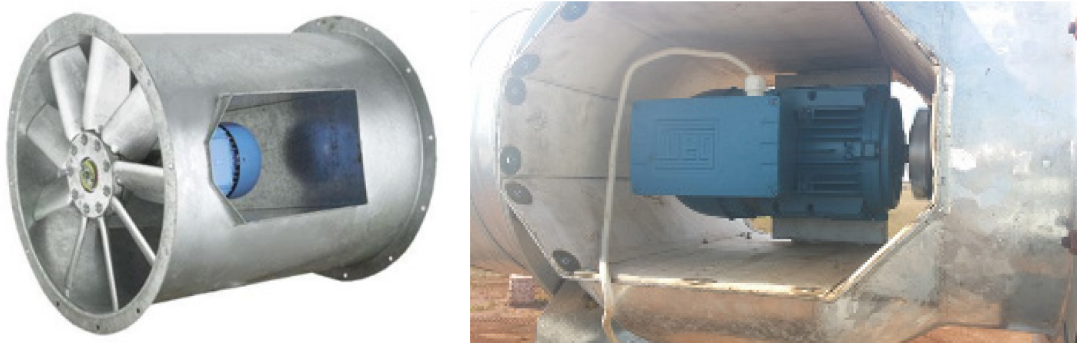
Figure 33: A typical Bifurcated Axial fan; and the 1.5 KW 2P 220V B3T WEG ALLY motored axial fan installed at the model kiln stack
