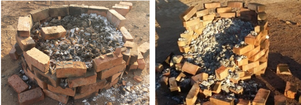
Figure 40: Typical 'fire-box' used for starting the brick firing process
