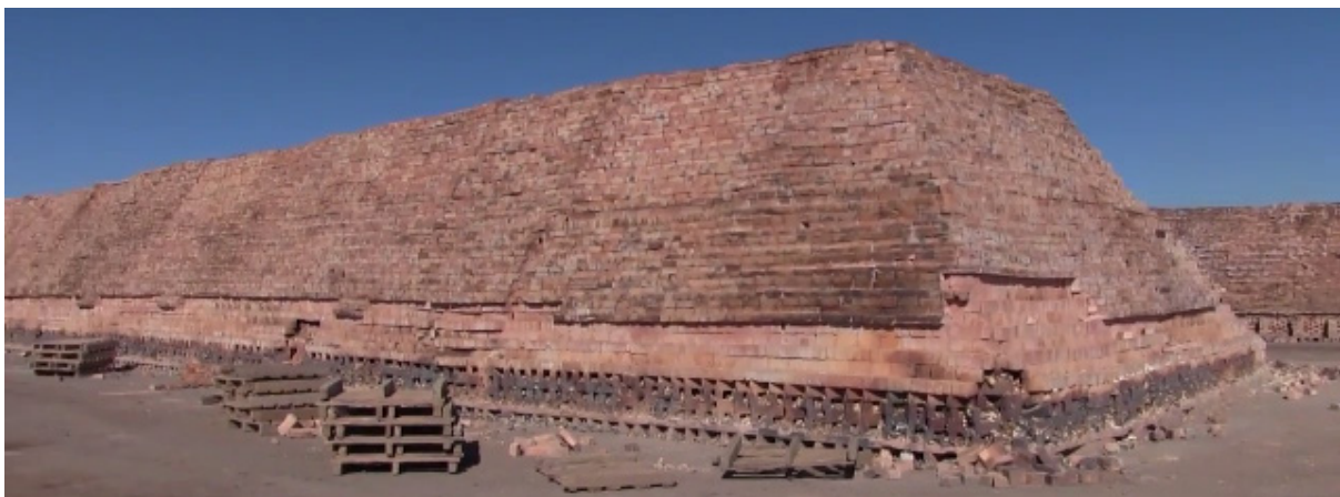
Figure 1: A typical clamp kiln at Nova Bricks, South Africa (NOTE: containment of emissions is not feasible)
