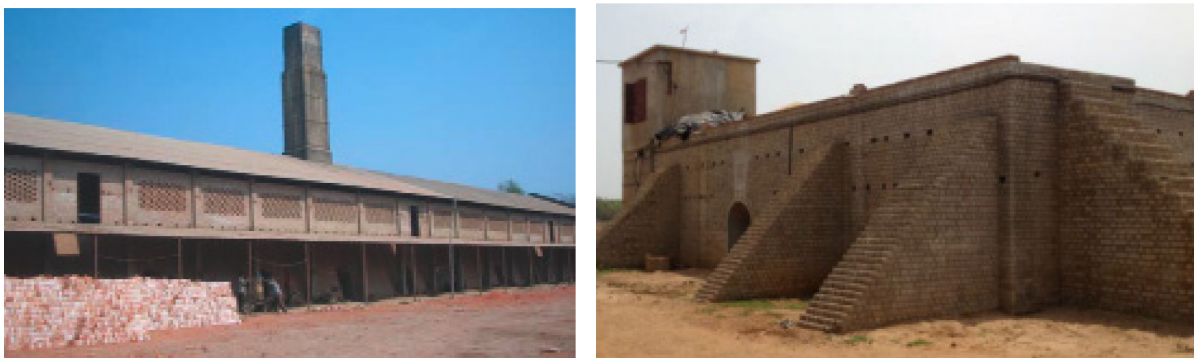
Figure 8: Hoffman kiln structures in Asia (Sarraf et al , 2011; Pradhan, 2015)
