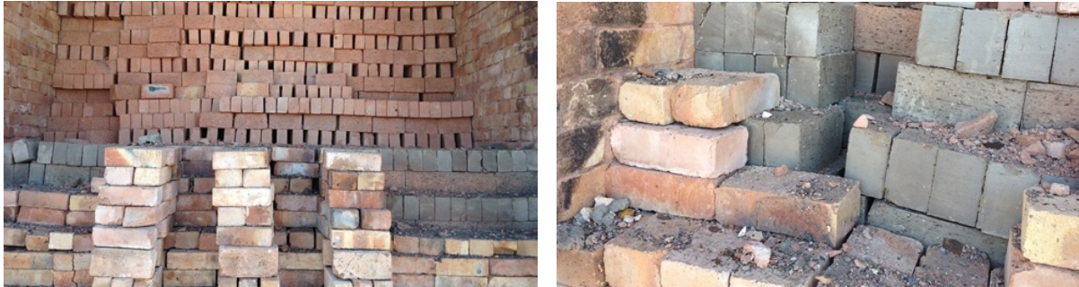
Figure 88: Cross section of model kiln firing chamber showing under-fired, partially fired and evenly fired bricks during unpacking from the northern side of the kiln (left); and under-fired bricks from the south side during unpacking of the kiln (right)
