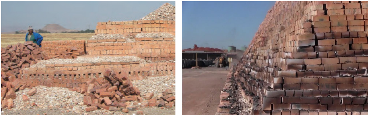
Figure 21: Brick and fuel packing methodology in informal (left, Cermalab (2014)) and formal clamp kiln (right, Nova Bricks, South Africa)
