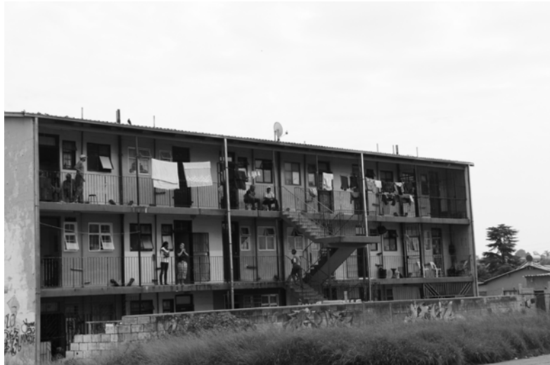
Fig 46 _ Housing Units (Author, 2017)
