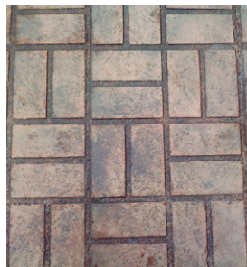
Figure8. 14 Basket brick paving pattern (Menarek Stamped Concrete 201)
