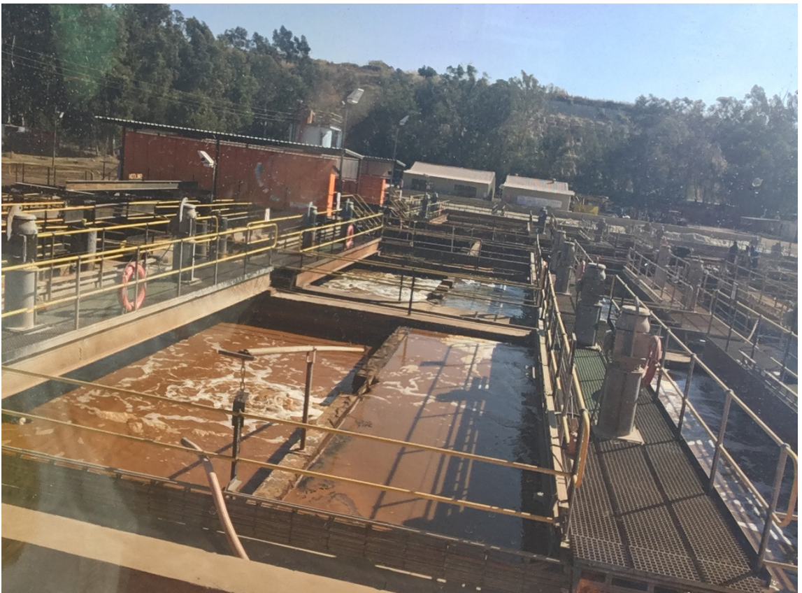
Figure 8.50 AMD treatment facility in West Rand (Author 2017)
