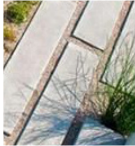
Figure8.13 Concrete blocks cast in situ (Pinterest 2017)
