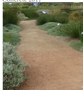
Figure8..15 Soil crete pathway in Green point park Cape Town (Author 2012)
