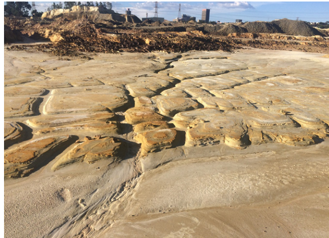
Figure3.6 Erosion caused by drainage (Author 2017)
