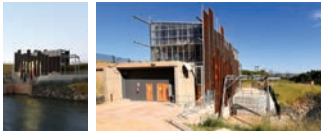
Fig_69b. Stortemelk Hydroelectric Plant (EWA 2016).
