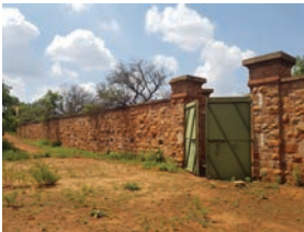
Fig. 63b. Fort entrance from interior (Author 2017).
