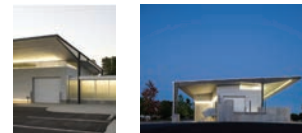
Fig_69l. Cox Communications Distribution Center (AchDaily 2016).
