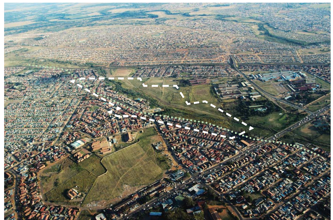
Figure 1.6 Right: Aerial view of site, southward view
