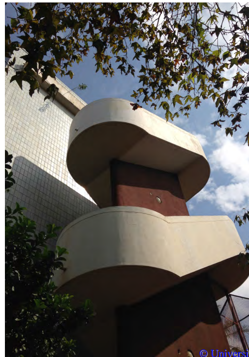
Figure 22: A-block exterior stairs.
