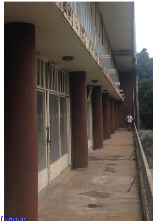
Figure 23: First floor balcony C-block.
