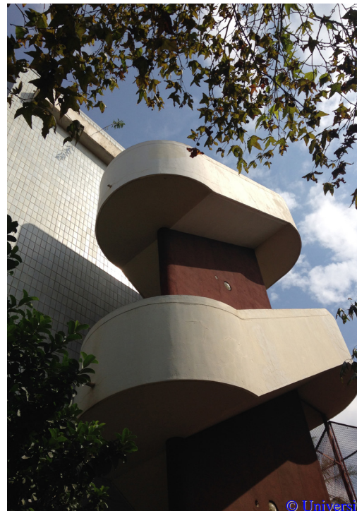
Figure 22: A-block exterior stairs.
