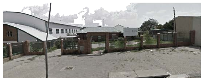
Fig.6.6: Community hall and nursery in Roberts avenue (Author, 2017)
