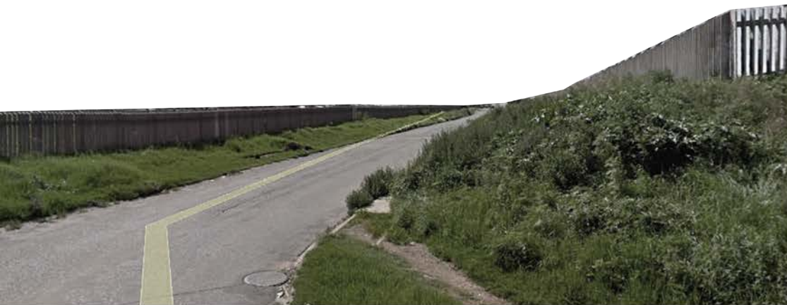
Fig.4.19: Image of concrete palisade fences(Author,2017)
