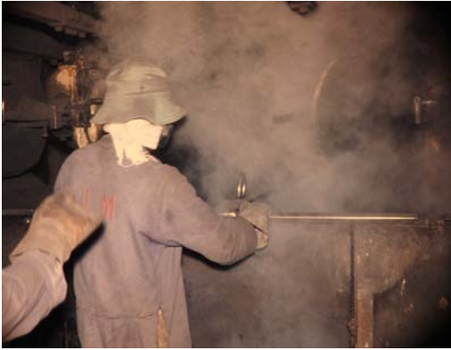
Figure 3.41. Positioning hopper without full PPE (FInsen, 1970's)
