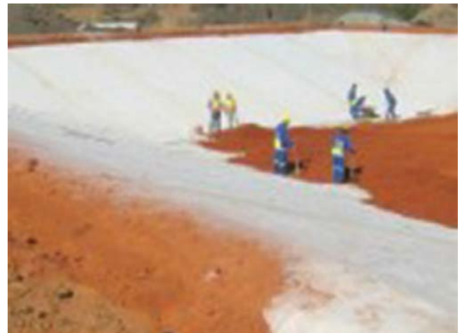
Fig 7.43. Geosynthetic clay liner - Envirofix (Kaytech.co.za, 2017)
