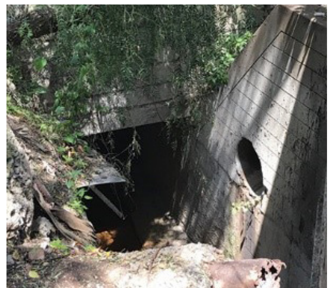
Fig 7.3. Spruit as concrete channel outlet (Author 2017)
