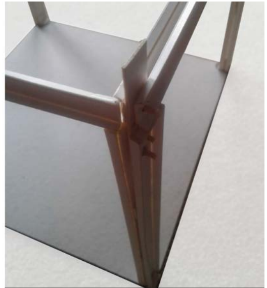
Figure 05.14.6 Detail view of steel plates serving as spacers and fixers in the structural elements
