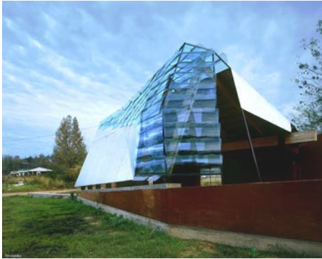
Figure 2.23: Glass Chappel by Rural studio, constructed from recycled windscreens. (Rural Studio 2000)
