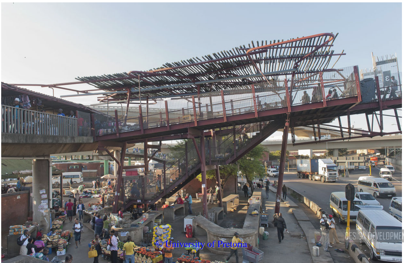
Figure 5.8: Warwick Junction bridge, acting as an architectural stent. (SAIA 2016)
