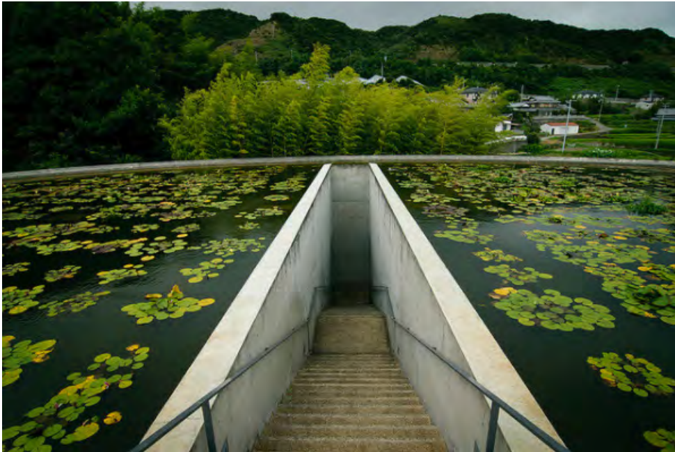
FIG 86 : Critical regionalism in action in the Water Temple in Awaki Island, Tadao Ando (Martin, 2013)
