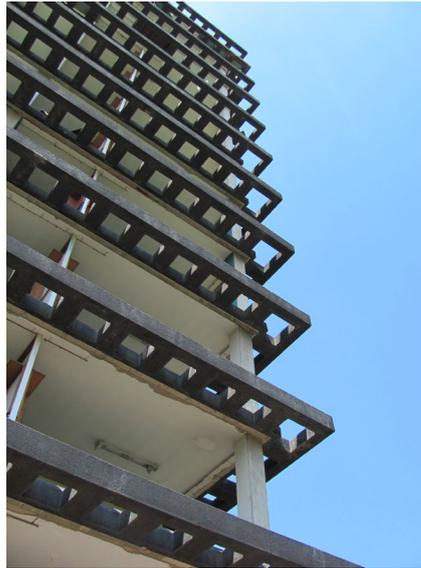
Figure 114 - View of brise soleil from ground level with framing pattern (by Author)
