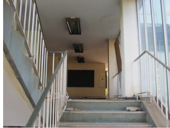
Figure 56 - View towards lift from main staircase (by Author)
