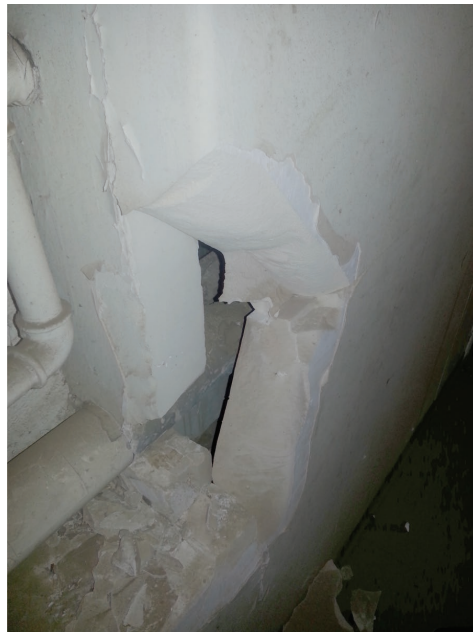
Figure 36 - Service shaft wall (by Author)
