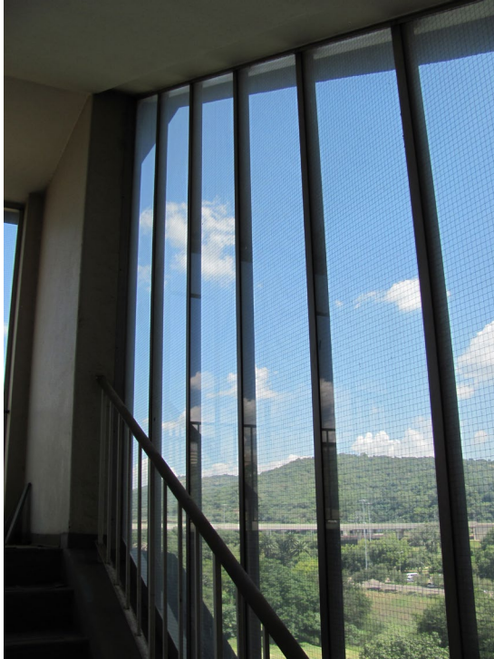
Figure 54 - Wired glazing on main staircase (by Author)
