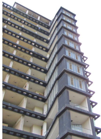
Figure 57 - View of main staircase from parking area (by Author)
