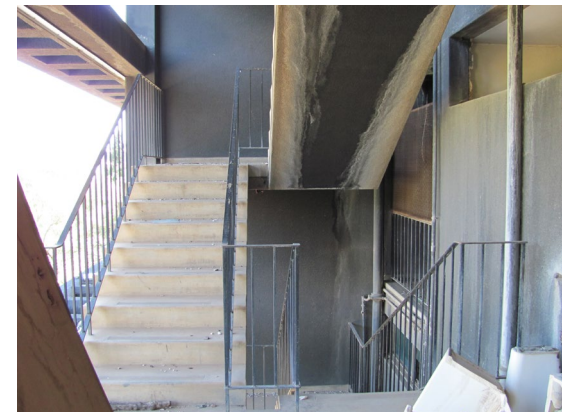
Figure 59 - View of fire escape from main circulation (by Author)
