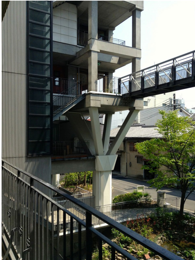
Figure 86 - The skeleton structure of the building is shown, with the more transient infill levels visible (Hiroshi Shoji Architects 2013)
