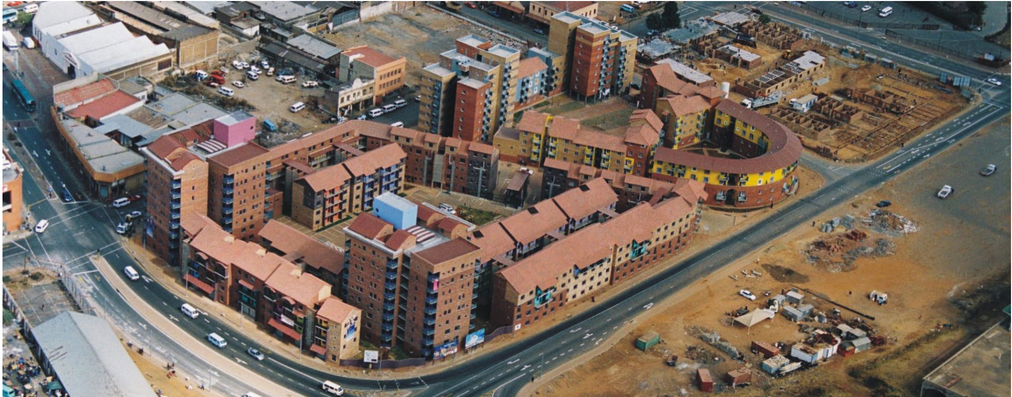
Figure 108 - Aerial view of development (Savage & Dodd 2005)
