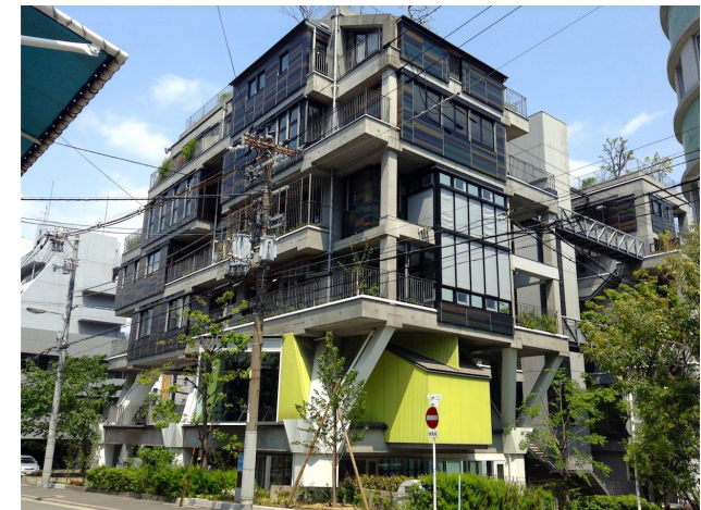
Figure 85 - Exterior of building from street level. Different facades and layouts can be seen, with the skeleton structure remaining constant throughout (P_kan 2013)
