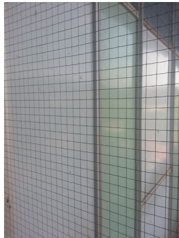
Figure 156 - Wired glass and green cladding panels (by Author)
