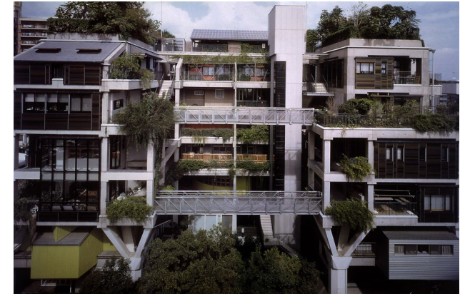
Figure 84 - View of building from adjacent buildings, indicating exposed and hidden walkways (Osaka Gas Company 1994)
