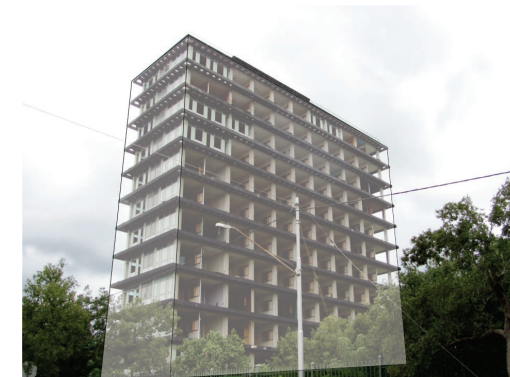
Figure 33 - Image emphasising the rectilinear shape of the building (by Author)
