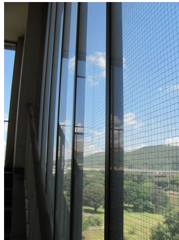
Figure 157 - Close-up view of wired glass in main stairway (by Author)
