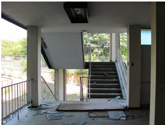
Figure 55 - View of main staircase from lift (by Author)
