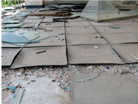
Figure 34 - Linoleum Flooring (by Author)
