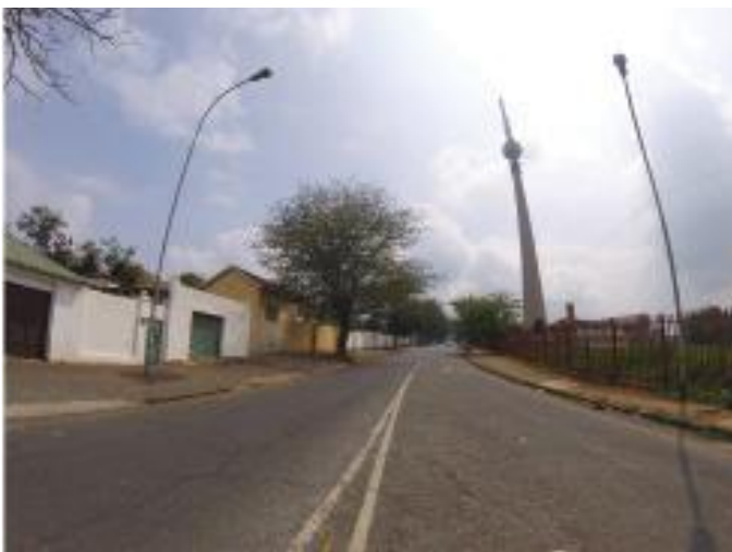
Fig 3.7 View of Semtech Tower from Symons road in the south
