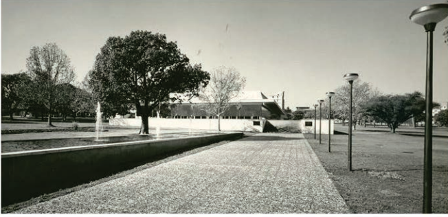
APPROACH TOWARD EASTERN SIDE OF THE MUSEUM PLINTH
