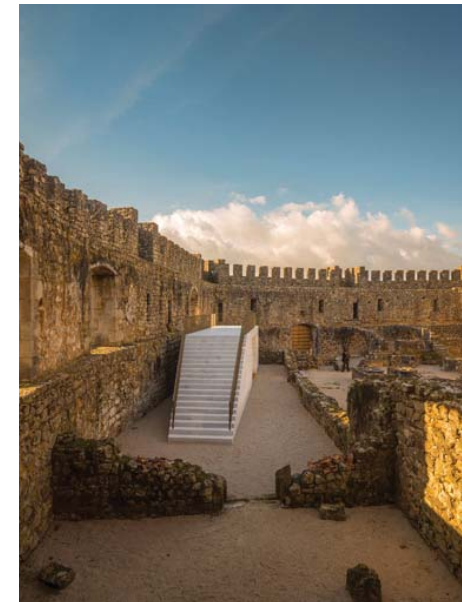
Fig.4.7 Photograph showing limestone monolith "staircase façade" (Guerra, 2014)
