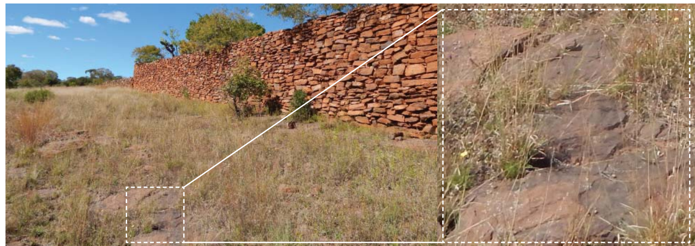
Fig.6.4 Photograph showing the site ground condition (Author, 2017)
