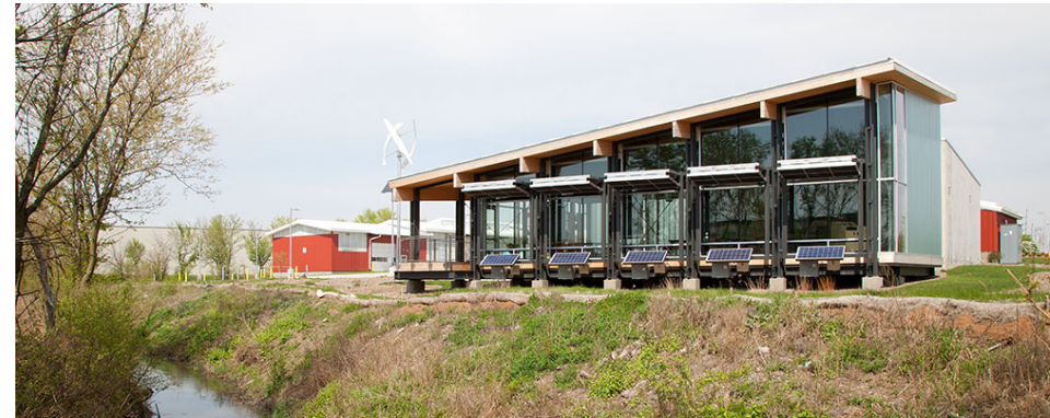
Figure 4.3.2 East Side Recycling Center main façade during the day (Shive Hattery, 2011)
