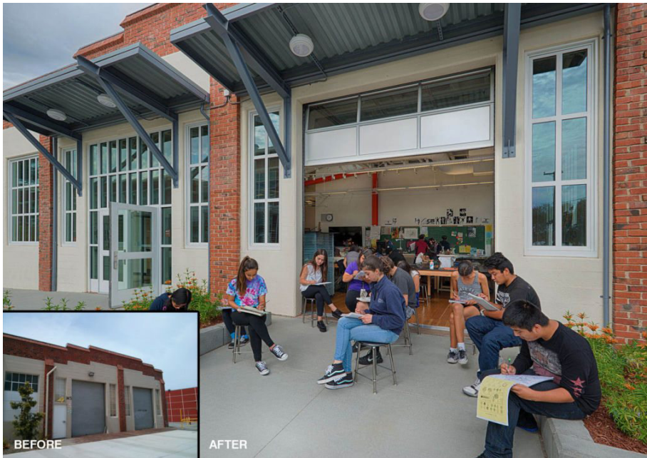
Figure 4.7.1 San Mateo High School exterior façade (AIA Redwood Empire, 2016)
