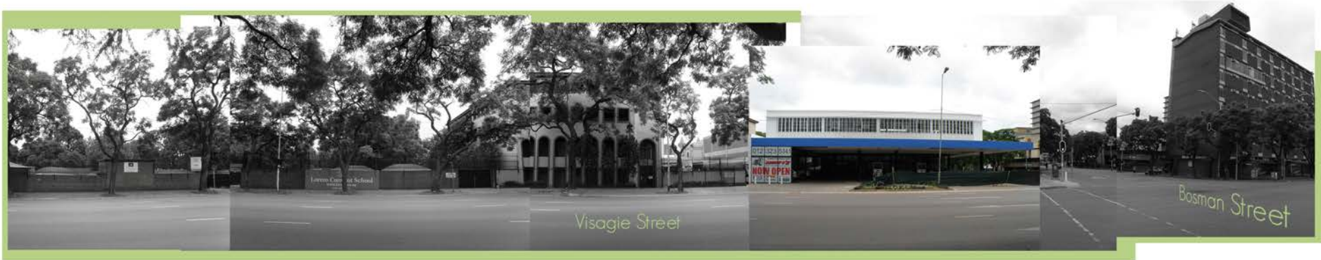
Figure 2.2.2.4 South elevation of adjacent buildings
