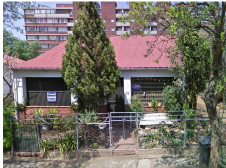
Figure 2.1.37: 15 and 17 Tulleken Street in 2009 (Google Earth 2017)
