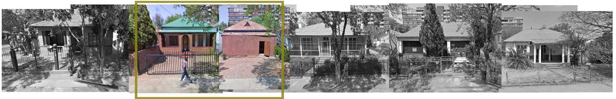
Figure 2.1.59: Tulleken Street elevation (Author 2017)
