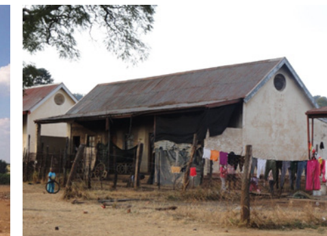
Figures 3.9d Illegal house
