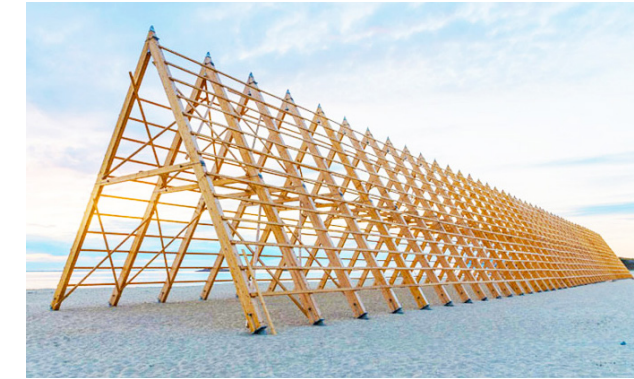
Figure 7.70 Repetition of timber structure
