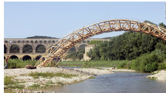
Figure 7.67 Context of bridge over water
