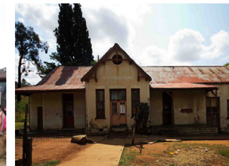
Figures 3.9e Dilapidated structure
