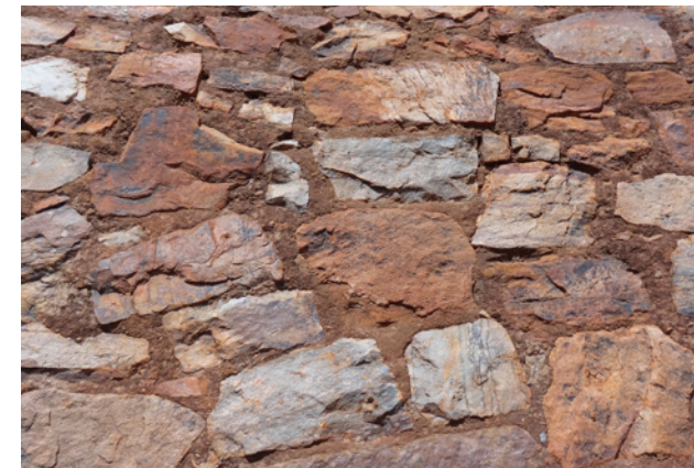
Figures 3.20d Irregular shaped local stone used in the building structure
