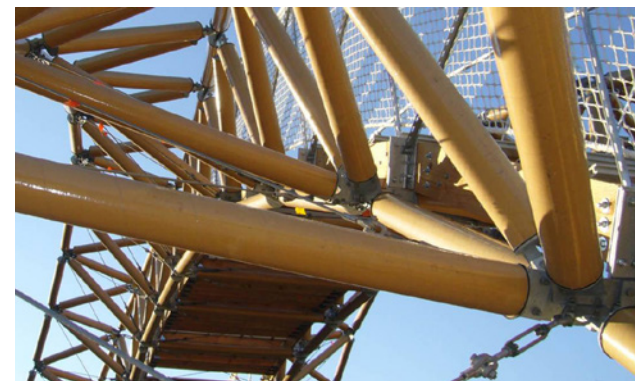
Figure 7.68 Steel modular joint system
