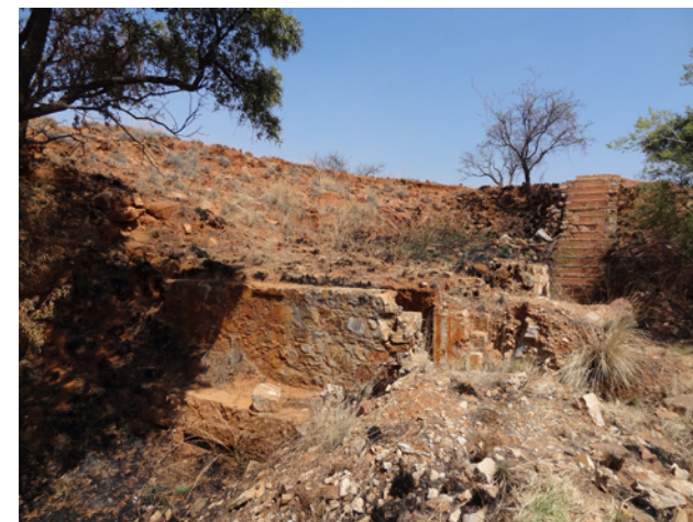
Figure 7.175 Fragility and damage to site
