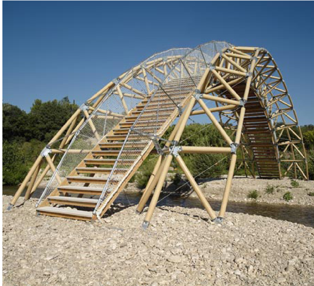
Figure 7.65 Shigeru Ban cardboard tube bridge 0152
