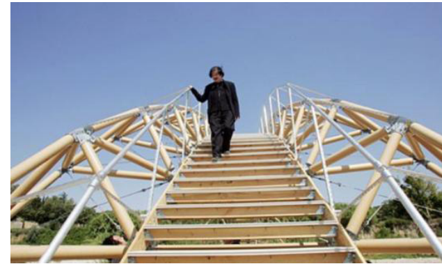
Figure 7.66 Stair structure of bridge
