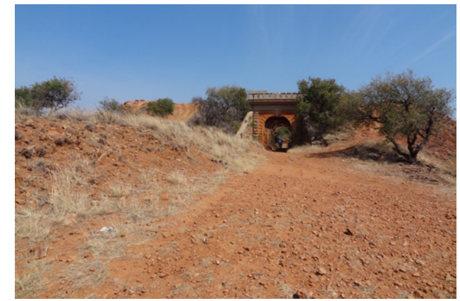
Figure 7.86 Approach to entrance
