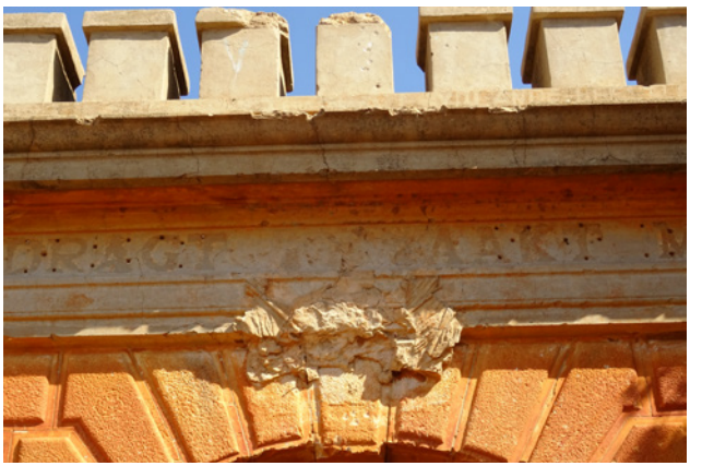
Figure 7.87 Detail of arch way
