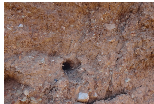
Figures 3.19f Local sand naturally compacted and exposed through erosion
