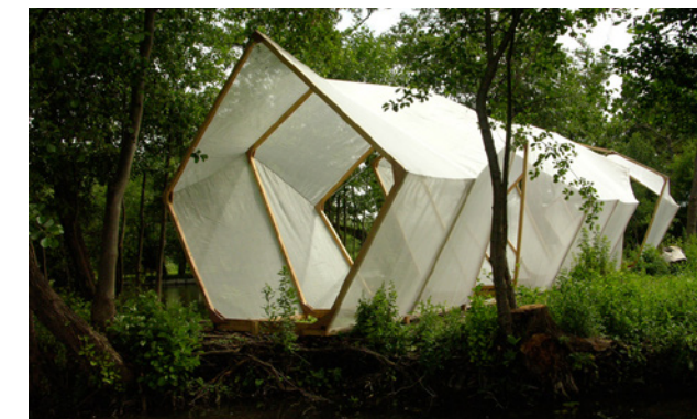
Figure 7.72 Timber and fabric structure
