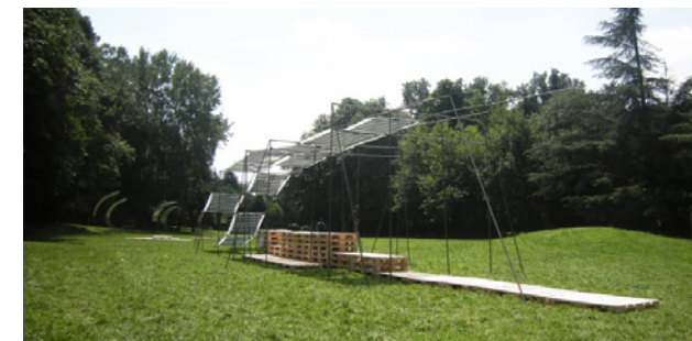
Figure 7.69 Steel roof structure over path
