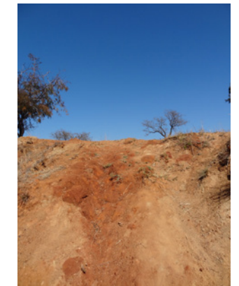
Figure 7.4 Photograph of slope August 2016
