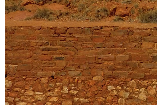
Figures 3.20c A structured construction of the local stone, used to build supporting walls
