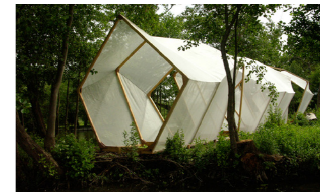
Figure 7.72 Timber and fabric structure
