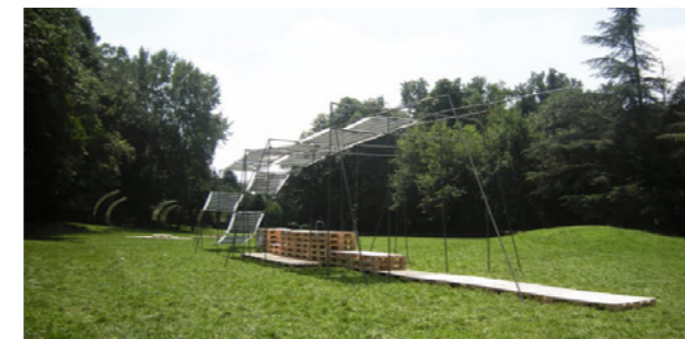
Figure 7.69 Steel roof structure over path
