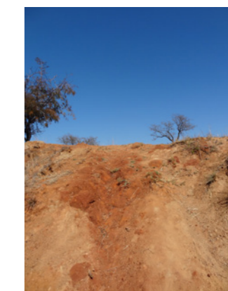
Figure 7.4 Photograph of slope August 2016
