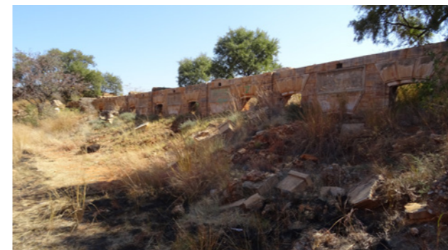
Figure 7.131 Overview of the rooms where the scene takes place
