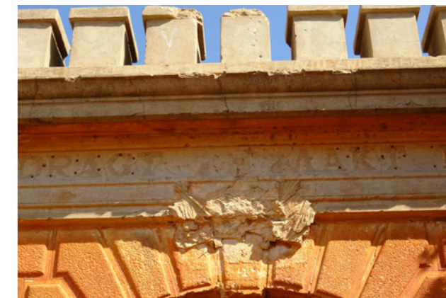
Figure 7.87 Detail of arch way
