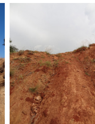
Figure 7.5 Photograph of slope July 2017
