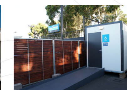
Figure 7.46 Portable disabled ablution block
