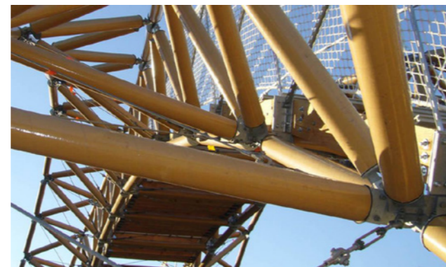
Figure 7.68 Steel modular joint system
