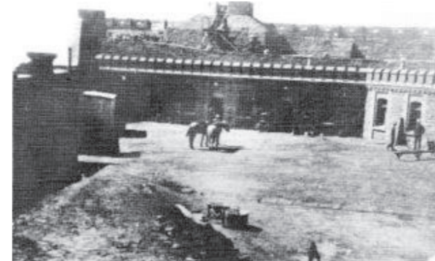
Figure 3.6b Original photo of Fort Schanskop courtyard
