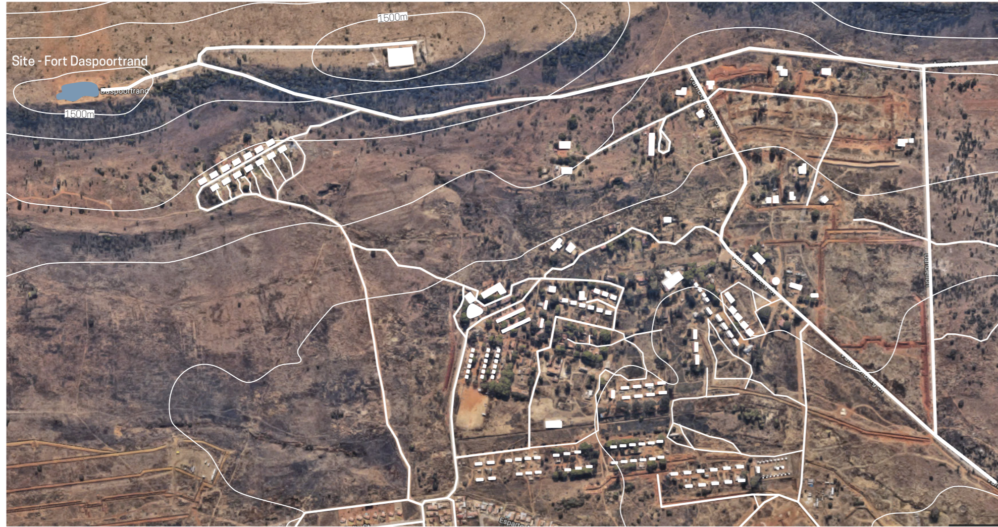
Figure 3.10 Aerial view of Fort Daspoortrand and Westfort Heritage Village
