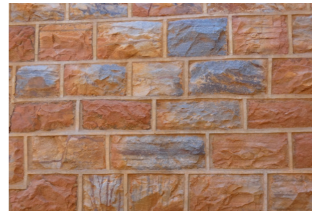
Figures 3.20a A construction of the local stone, detailed with a cement finish, used to build the majority of the fort
