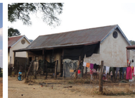
Figures 3.9d Illegal house
