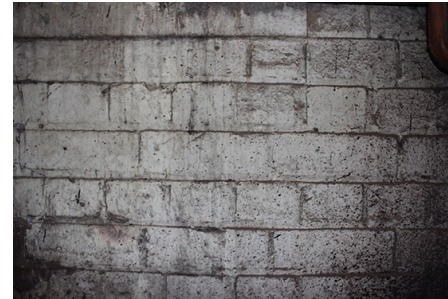
White washed clay bricks
