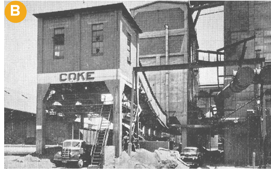
Figure 3.5: Coke screening & loading plant (City of Johannesburg Gas Department 1950)
