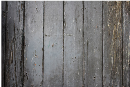
Weathered timber doors
