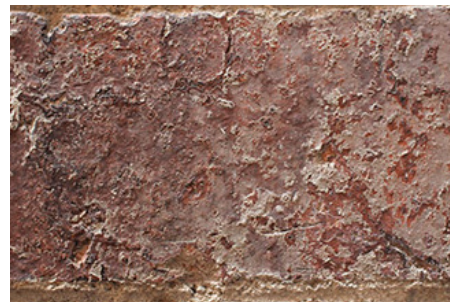
Weathered clay bricks
