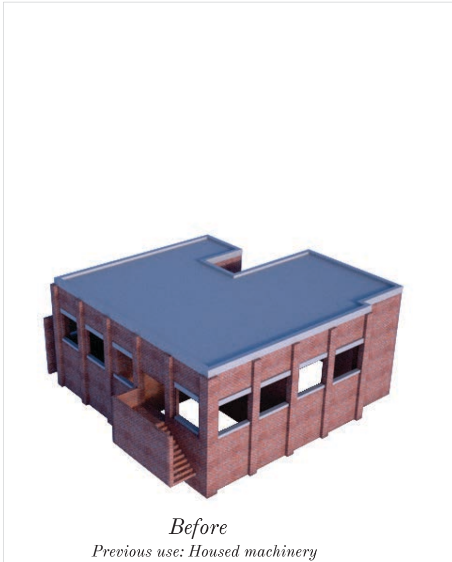
Figure 6.40: Power house before intervention (Author 2017)
