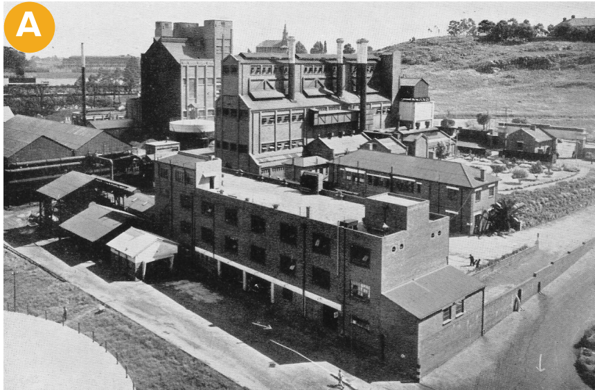
Figure 3.4: View from gasholder towards retort 1 & 2 (City of Johannesburg Gas Department 1950's)
