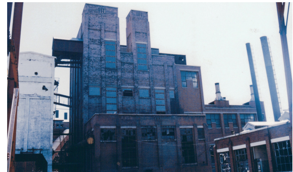
Figure 3.12: Coke grading & storage, Retort 2 and power house (Peter Finsen 1990s, edited by Author)
