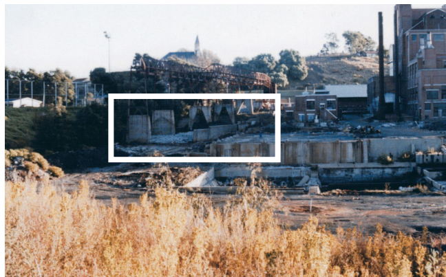
Figure 3.57: 1992 Partial demolition (Peter Finsen 1992, edited by Author)
