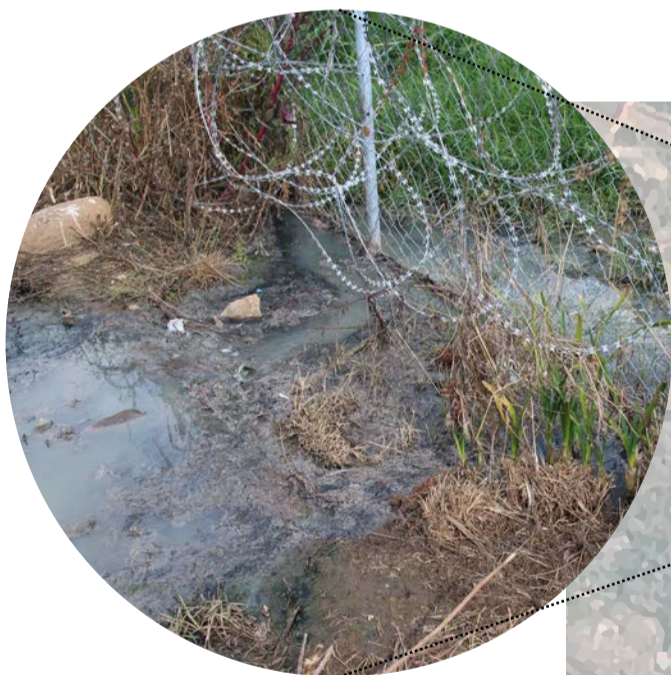
SEWAGE LEAKAGE AND SLIME DAM WATER MIXING
