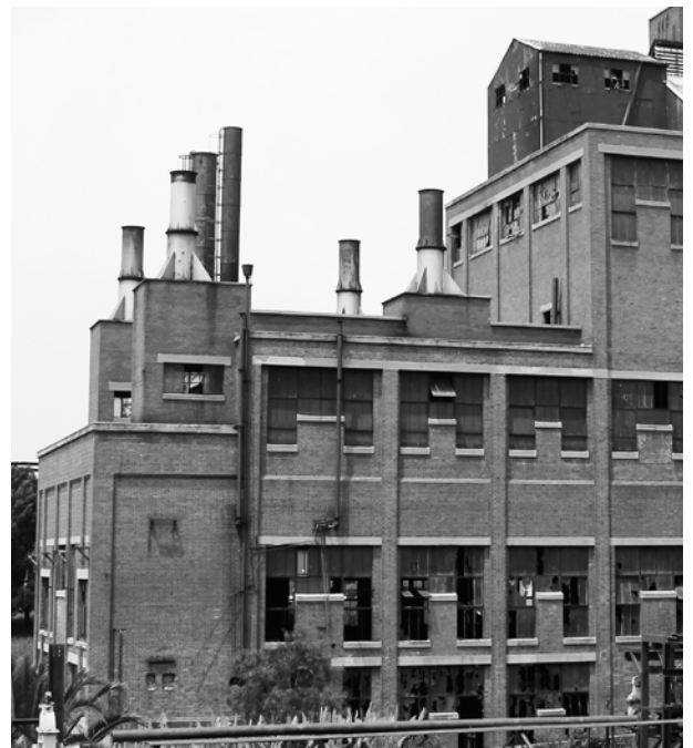
Figure 123 Chimney towers, the relationship between openings and structure (Photograph by Author, 2017)
