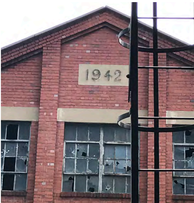
Figure 124 Brick eave detailing (Photograph by Author, 2017)
