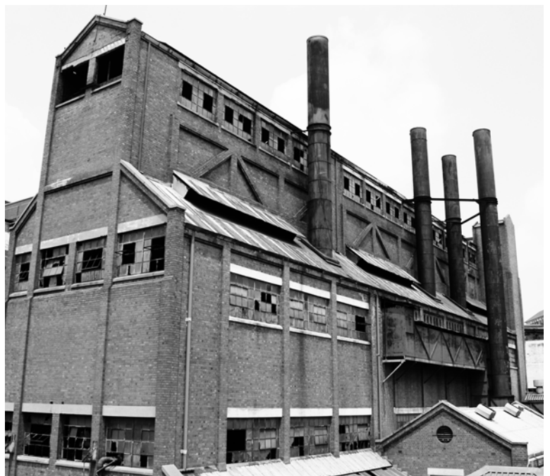
Figure 125 Chimney flues of Retort 1 (Photograph by Author, 2017)
