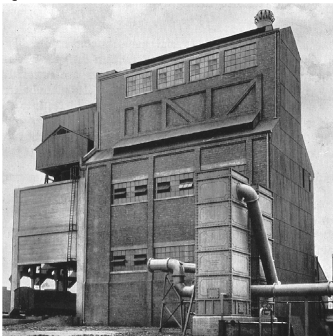
Figure 119 South-eastern facade of Retort No. 1
