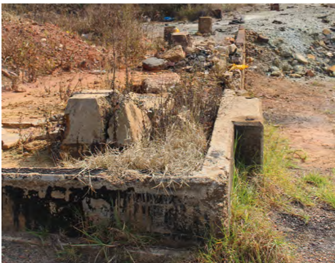
Figure 83 Column stubs (Photograph by Author, 2017)
