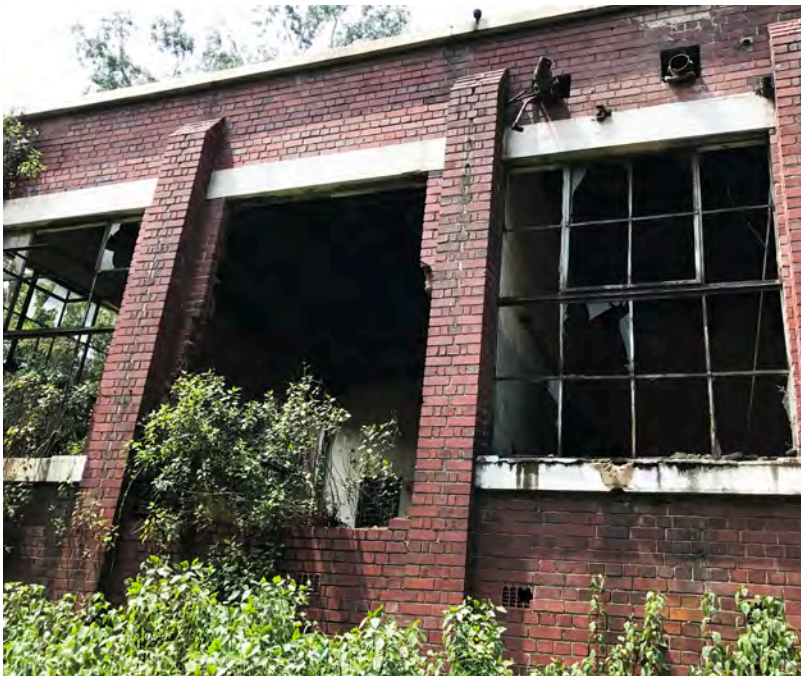
Figure 122 Concrete detailing around openings and structural expression (Photograph by Author, 2017)
