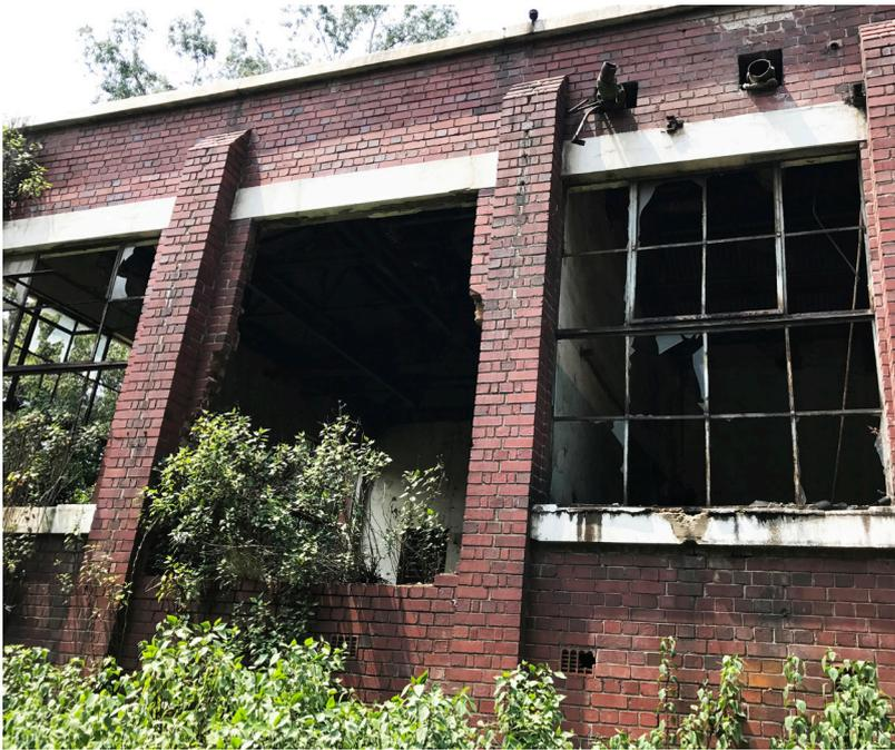
**Figure 122** Concrete detailing around openings and structural expression (Photograph by Author, 2017)
