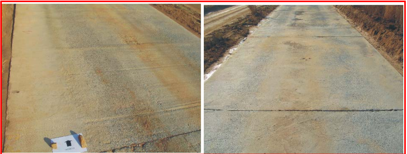
Figure 5: The surface of the SFRC slabs of section 2
