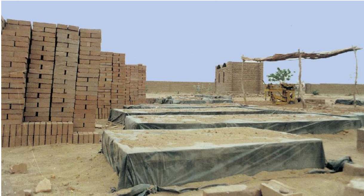
Figure 2.14: A curing process of compressed earth bricks
