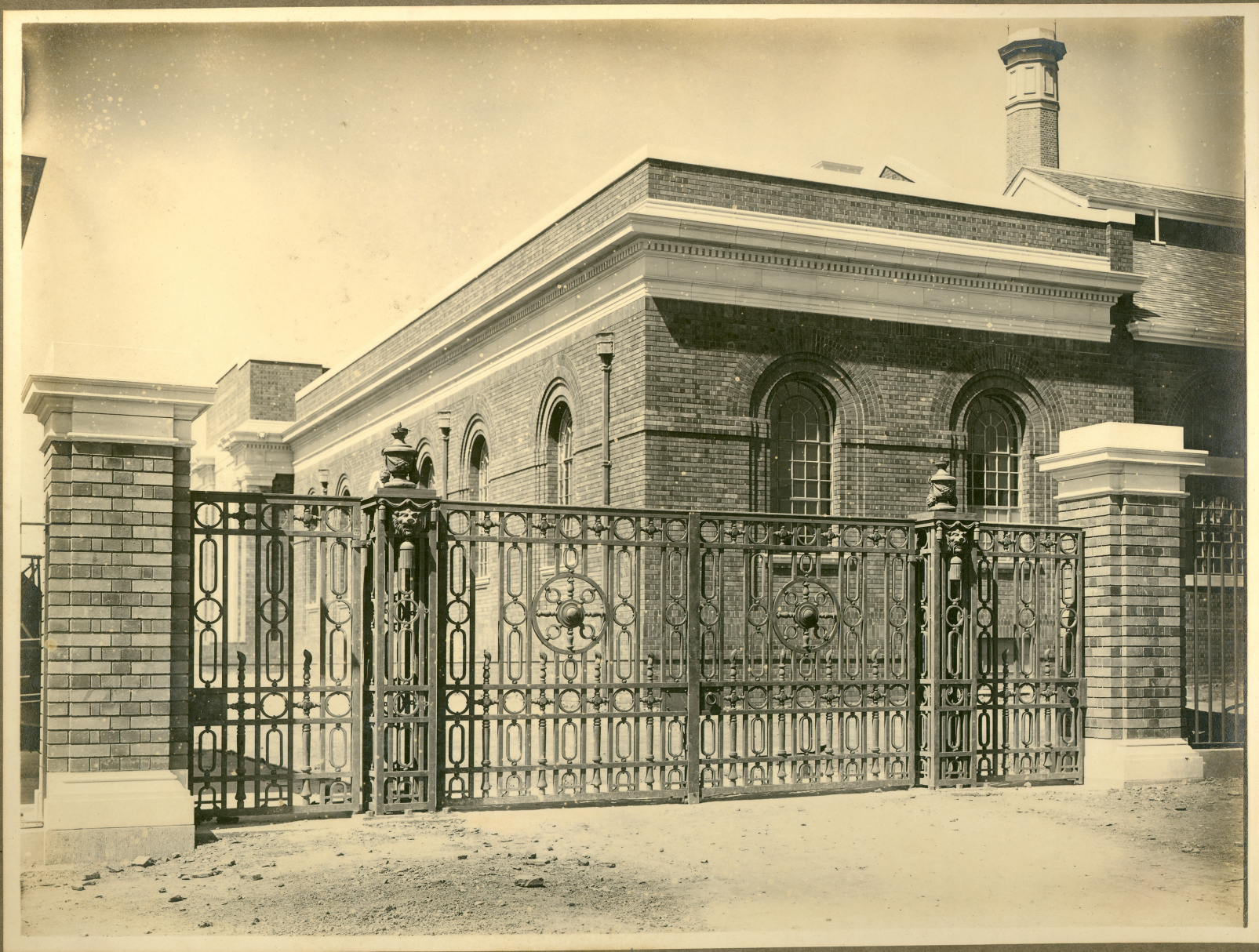
Building from Main Entrance Gateway
