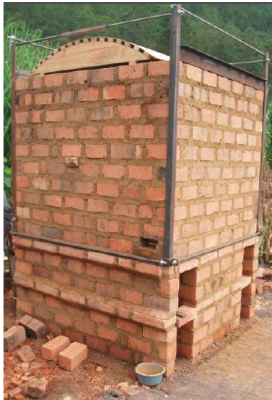
Figure 4.15: Kiln Constructed for Larger Clay Pots
